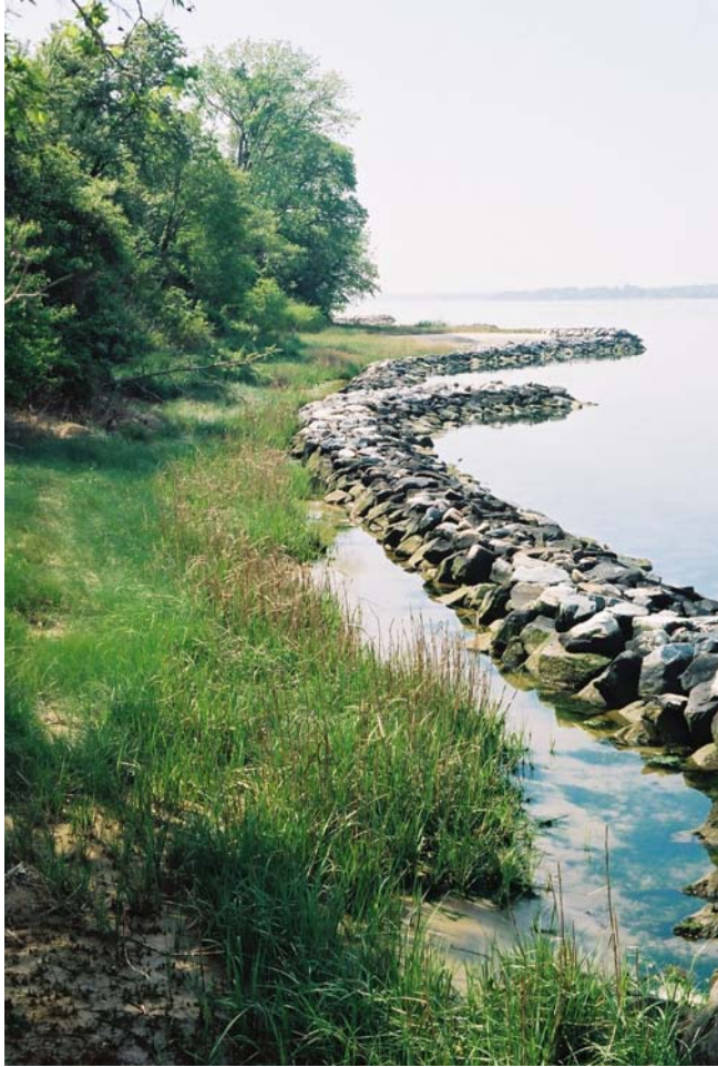
Figure . JP Park, Station 28+11
