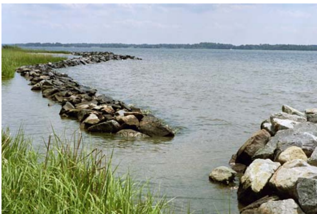
Figure . JP Park, Station 28+11, sill window
