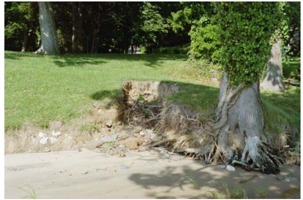
Figure . Epping Forest, Section 2, bank erosion
