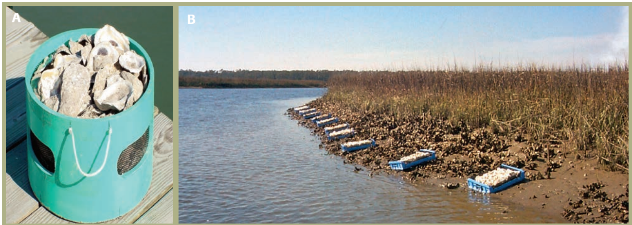
Figure 27. (a) Substrate baskets containing oyster shell prior to deployment. (b) Shell trays deployed on a fringing reef.
