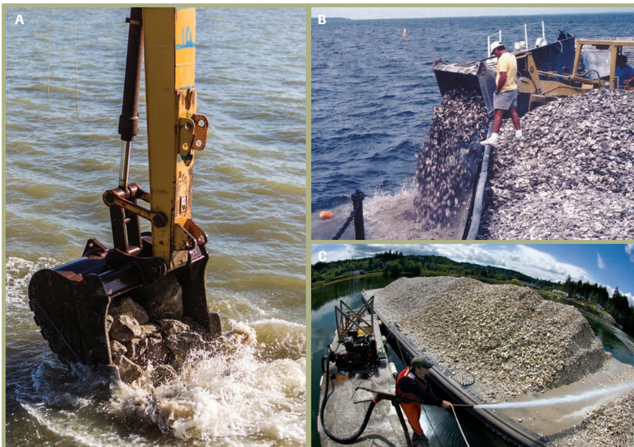
Figure 5A, B and C. (A) Limestone marl being placed as reef substrate in Matagorda Bay, Texas. (B) NC DMF vessel delivering marl to restoration sites. (C) Using a water cannon to spread oyster cultch over a restoration site in Dogfish Bay, WA.
